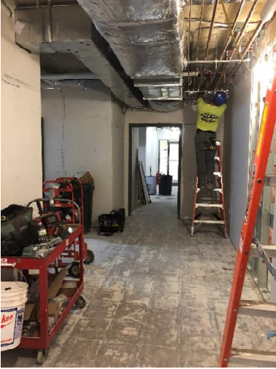
The photos above depict the new Outpatient area. The left photo is looking west down the hall, the center photo is the nurse station, and the right photo is the registrar area. The next step of construction is to tape and finish the walls so they are ready for paint.
