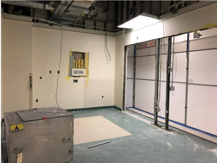
The three photos above depict the ER Nurse Station phase of construction. Demolition is nearly complete in this area. Stud wall framing of the new space will be ready to begin.
