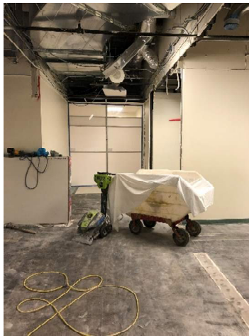
The three photos above depict the ER Nurse Station phase of construction. Demolition is nearly complete in this area. Stud wall framing of the new space will be ready to begin.
