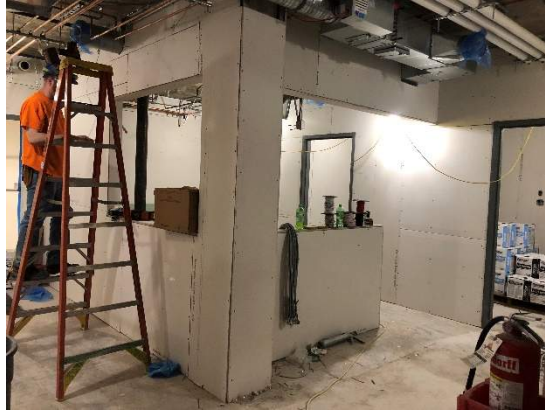
The photos above depict the new Outpatient area. The left photo is looking west down the hall, the center photo is the nurse station, and the right photo is the registrar area. The next step of construction is to tape and finish the walls so they are ready for paint.
