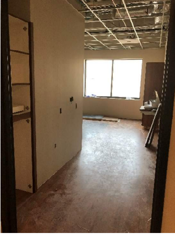
Various views of the progress taking place in the upper level Clinic / Med Surge addition. The nurse servers are being installed as well as the flooring. The final items to be completed is trimming out the MEPs, floor base, and dropping ceiling tiles.
